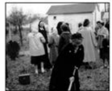
1958 Ground Breaking for Convent at Holy Family
